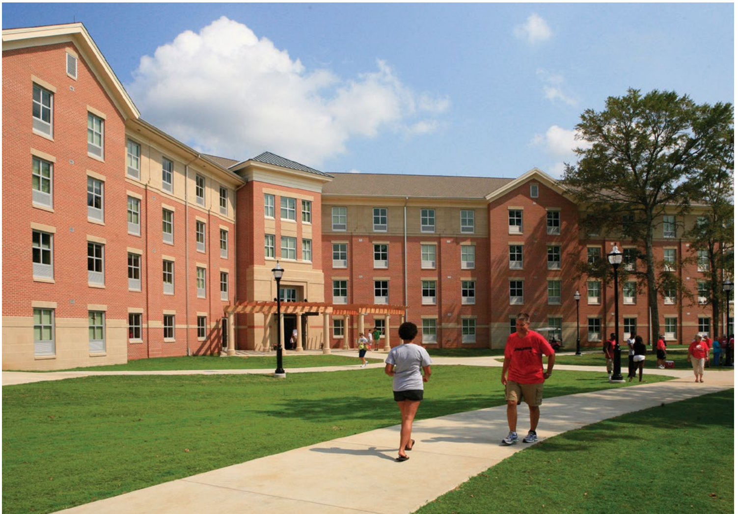
Stokes Hall, which has 330 beds along with classroom space and group study areas, has become a model for on-campus residence hall construction.
