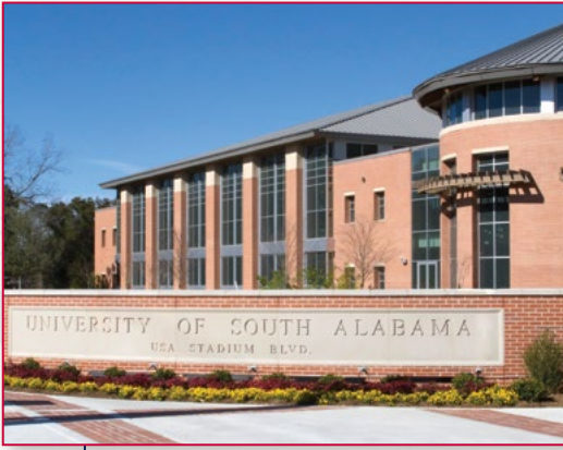
Completion of new campus entry portals.
